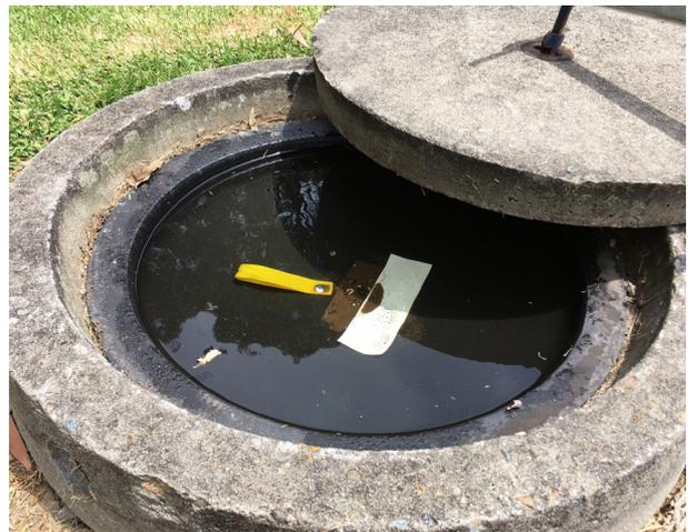
Leaking manhole covers are a major contributor to rainfall induced inflow. Sewer evaluation studies indicate that a typical manhole casting will allow an inflow rate from .70 to over 20 Litres per minute during rainfall occurrences.
