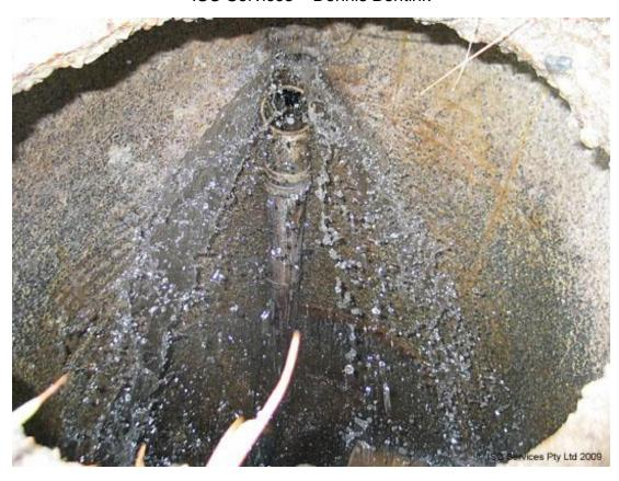
1. Infi-Shield Gator Wrap. Joint failure can occur due to ground settling, expansion and contraction of soils, vibration and damage to new structures and poor construction or missing butyl rope. Prevention is better than repair and externally Gator Wrap-ping all new precast concrete joints in manholes, pump stations and pits is easy to see and a simple yet valuable long term investment in preventing premature joint failure.
