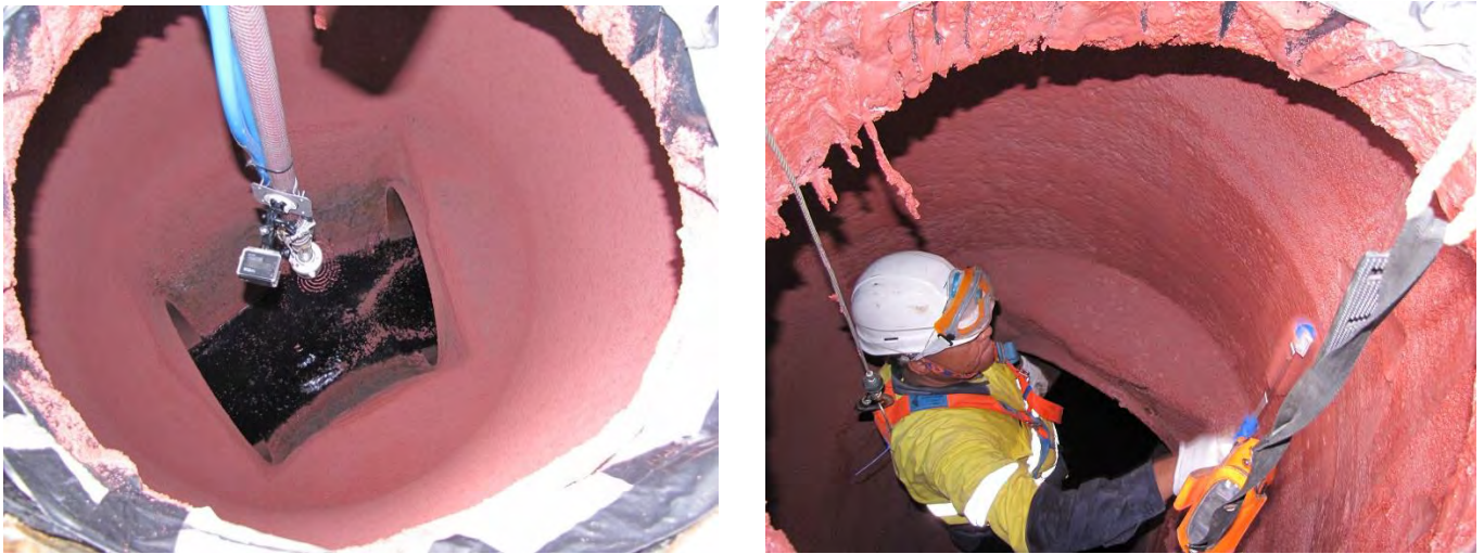
Figures 9 &10 - Spin Casting and roller finishing
