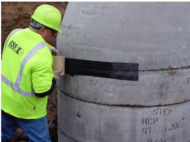
Preventing the development of I/I is the simplest and best approach for new structures being constructed and includes the use of quality, well proven components, appropriate design and good installation techniques. Simple innovative approaches such as a flexible high-quality external wrap for precast joints to ensure that movement of joints does not result in failure will help cost effectively prevent early development of leaks.
