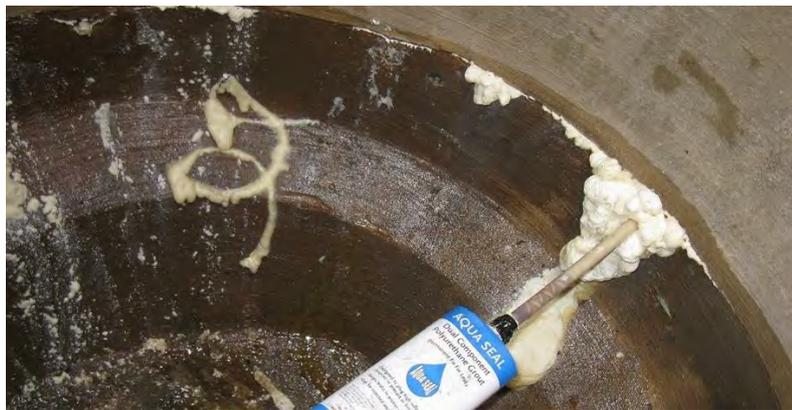
Where a high rate leak is occurring at a pipe or maintenance hole joint or crack, this can be quickly stopped through use of a made for purpose fast acting polyurethane foam.
