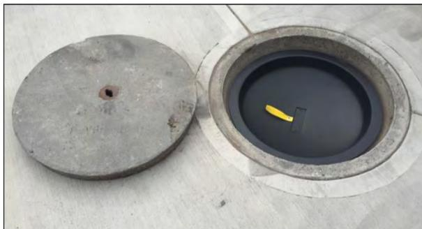
MH Insert/ inflow dishes are a simple and easy method to prevent rainwater flowing in through lids and frames during rain events.
