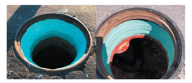
An inexpensive and permanent method of sealing the grade adjustment ring area and joint sections in a manhole or catch basin from inside of the structure. This state-of-the-art urethane material is easily applied by certified installers.
