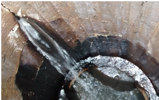
INFILTRATION LEAK
