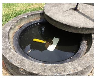
Leaking manhole covers are a major contributor to rainfall induced inflow. Sewer evaluation studies indicate that a typical manhole casting will allow an inflow rate from .70 to over 20 Litres per minute during rainfall occurrences.
