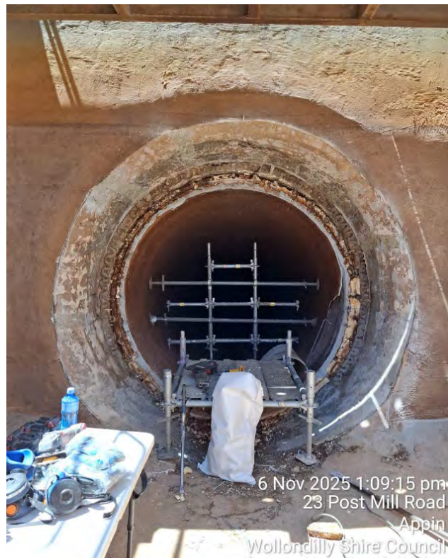
Figure 3 Surface preparation Nov 2025 Photo Courtesy of Interflow
