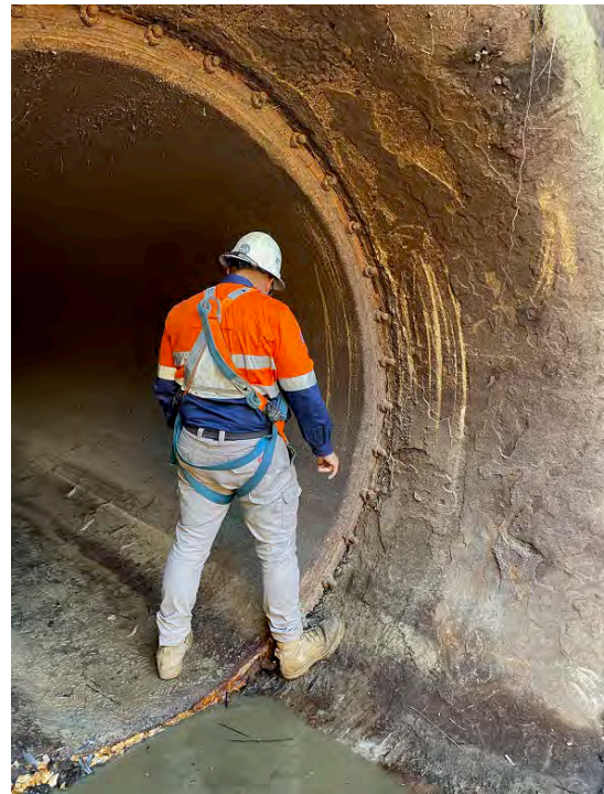
Figure 1 Inspection of Joint before HydraTite installation, April 2023
