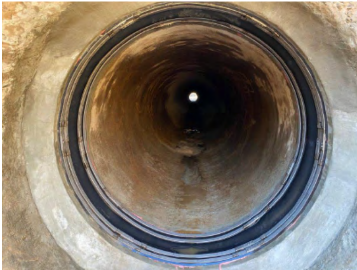
Figure 2 April 2023 Completed Job, Photo Courtesy of Interflow
