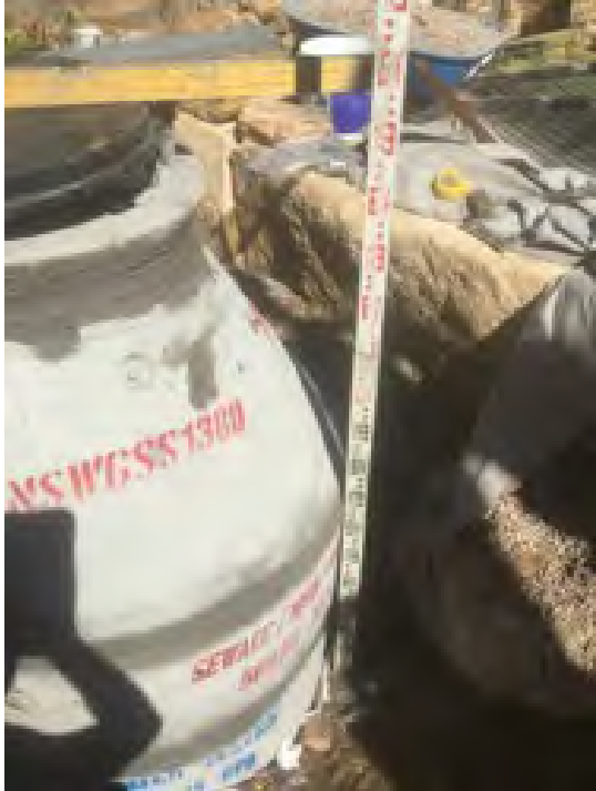
Figure 1 Common manhole installation, mortar joints
