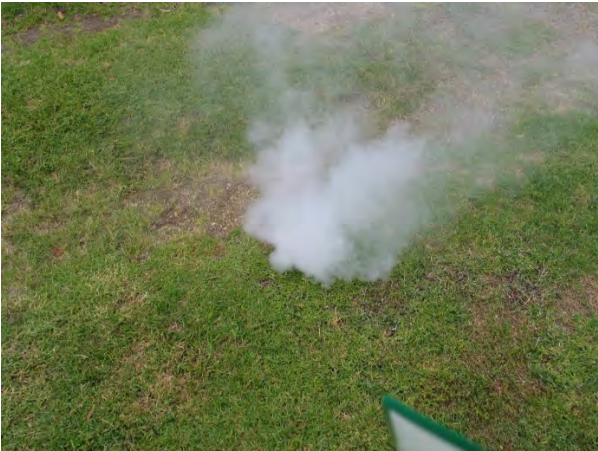
Figure 10 Smoke from the ground, likely a damaged pipe allowing infiltration
