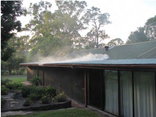
Figure 9 Smoke from a Roof Vent – correctly operating and not a defect
