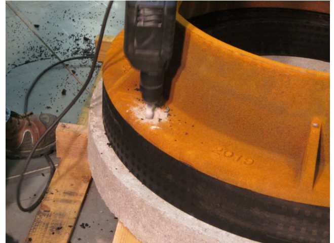
2. With the required amount of rings and frame in place, use the masonry drill bit and hammer drill to drill through the PRO-RING into the top of the manhole cone or flat top.
