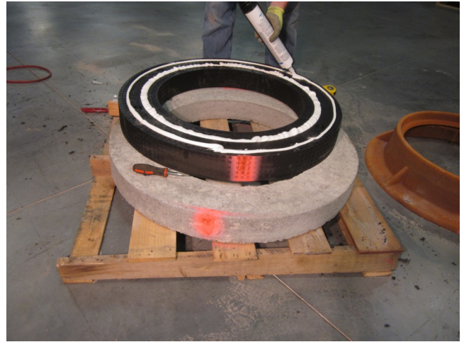
8. Overfill the two grooves in the underside of the Grade Ring with M-1 Adhesive. Be sure to place some extra adhesive around each of the drilled holes.
