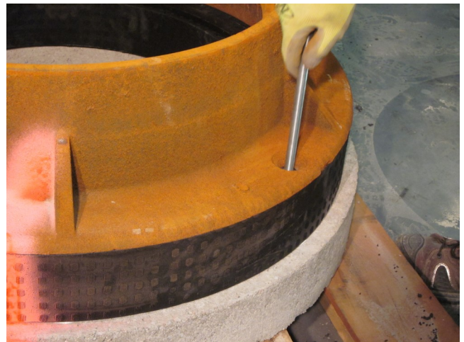
12. If using concrete anchoring adhesive, place the threaded rod into each of the previously drill holes and let the adhesive cure prior to installing the washers and nuts.
