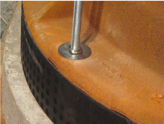
15. Place a large flat washer or fender washer, lock washer and nut onto each of the threaded rods.
