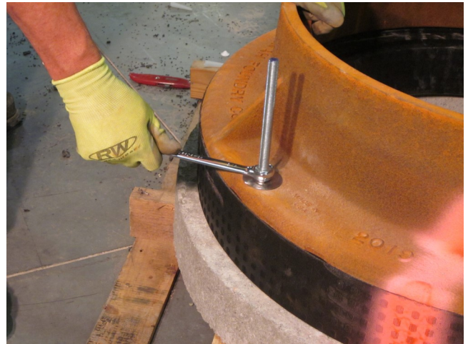
16. Tighten the nuts on each of the threaded rods.
