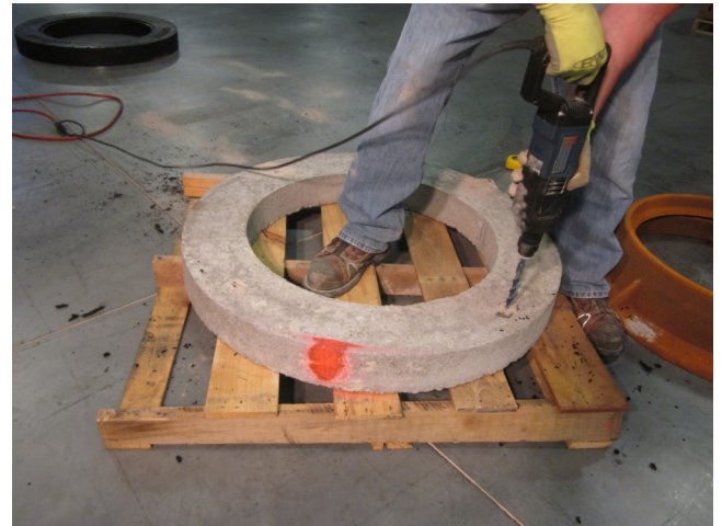
4. If necessary, finish drilling the holes in the top of the manhole cone or flat top to the required depth for either drop in anchors or concrete anchoring adhesive.
