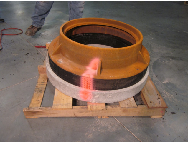
11. Place adhesive on the top of the Finish or Angle Ring and then install the manhole frame making sure to align with the previously applied marks so the holes line up.
