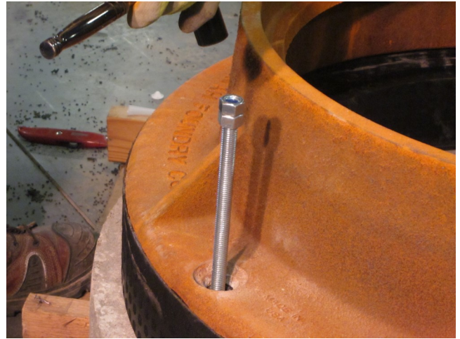
14. Using a double nut, tighten the threaded rod into the internally threaded drop in anchor until tight.
