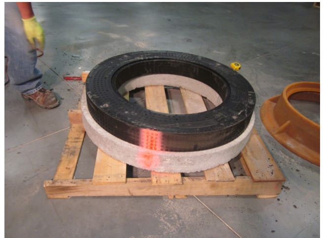
10. Flip the ring with the adhesive side down onto the manhole making sure to align with the previously applied marks to ensure the holes will line up.
