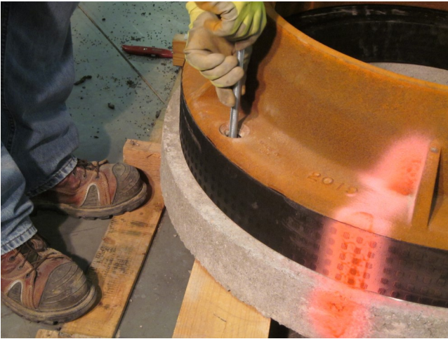
13. If using the internally threaded drop in anchors, position and start threading the rod into the anchor until finger tight.
