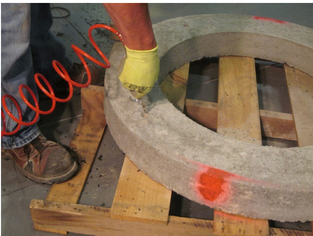
5. Be sure to remove all of the concrete dust and debris from the anchoring holes using compressed air.
