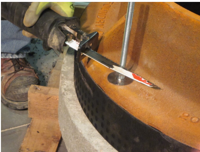
17. Using a reciprocating saw, hack saw or cutoff wheel, cut off any excess threaded rod and discard.
