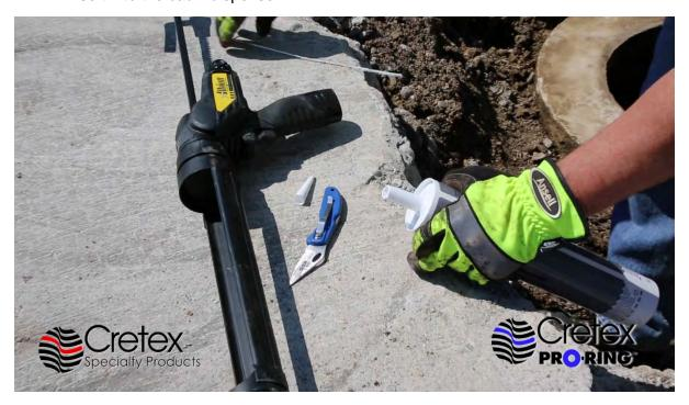
9. Apply a heavy bead of caulk to both the inner deep groove and the outer shallow groove of the grade ring. Make sure the adhesive protrudes beyond the surface of the ring to allow proper adhesion and sealing to the cone.
