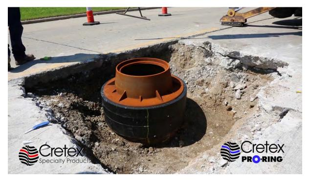
22. At this point the installation of Cretex Pro-Ring<sup>™</sup> is complete and the excavation can be backfilled immediately.
